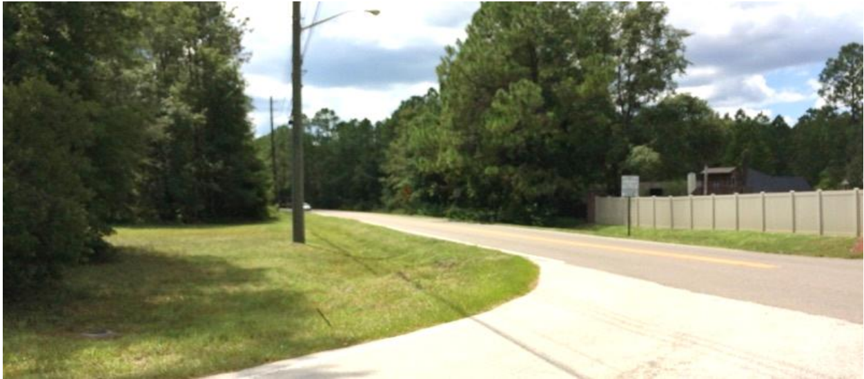
The subject site on the left facing south along Old Middleburg Rd S. at the Hipps Rd./Old Middleburg Rd. S. intersection
